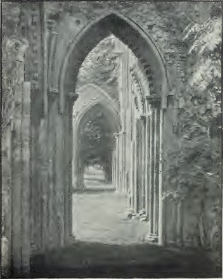
VIEW THROUGH CHOIR LOOKING SOUTH.
